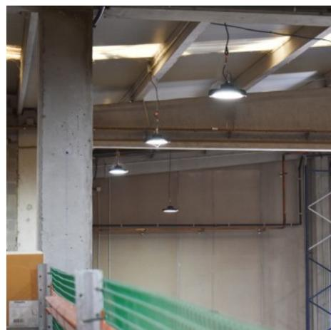
**Campana LED industriale - Driver LIFUD - 150W - 160lm/W - Chip PHILIPS - Dimmerabile 1-10V - IP65**
